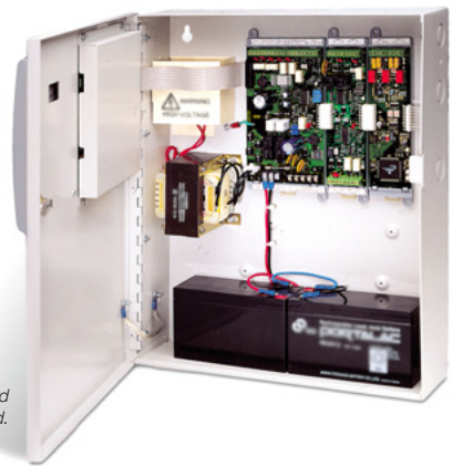
Cabinet with option card and batteries installed.
