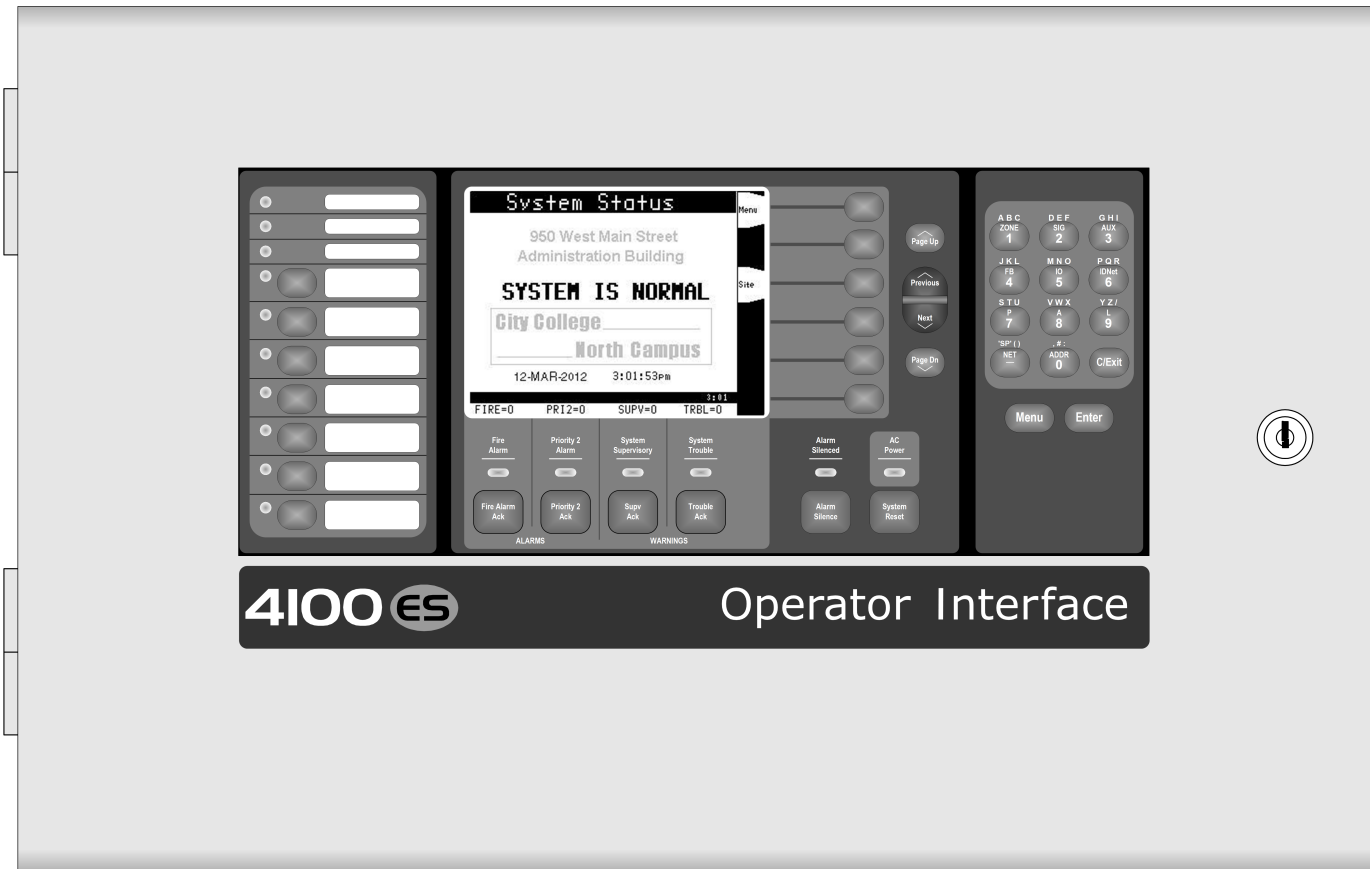
Figure 11: Remote InfoAlarm Command Center Front View
